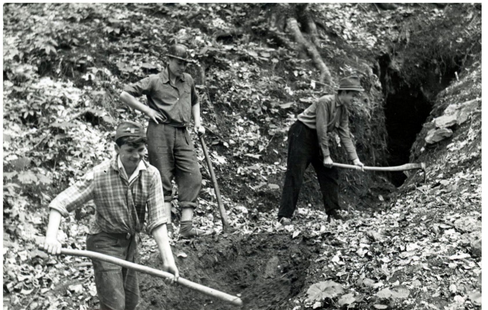
Works in front of the shaft of the second French mine 1959 / MGZ
