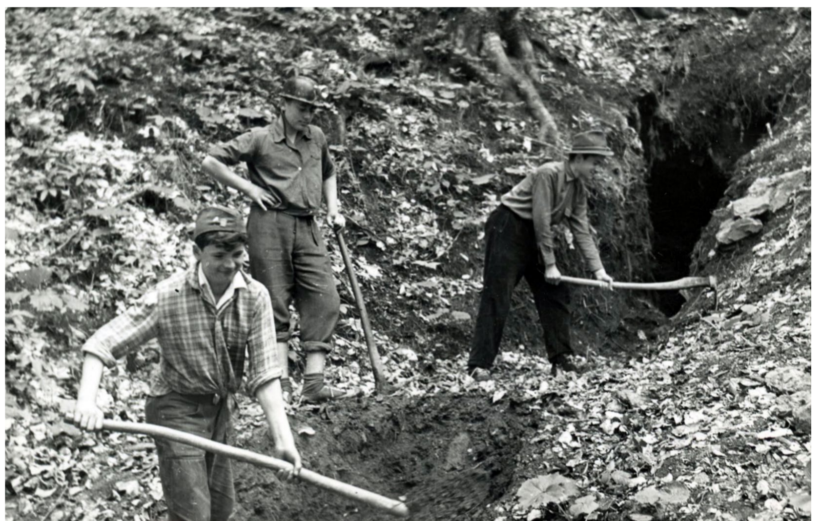
Works in front of the shaft of the second French mine 1959 / MGZ
